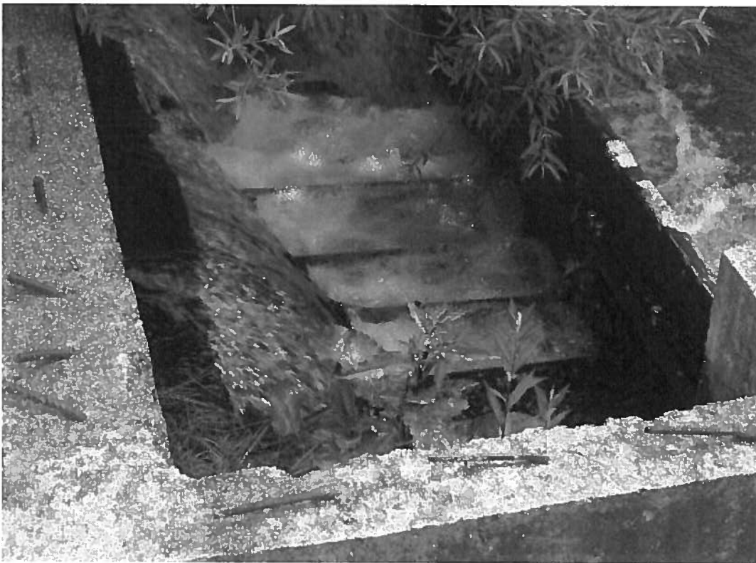
Figure 37. This rebar is bent to a horizontal position to help prevent impalement of farm
