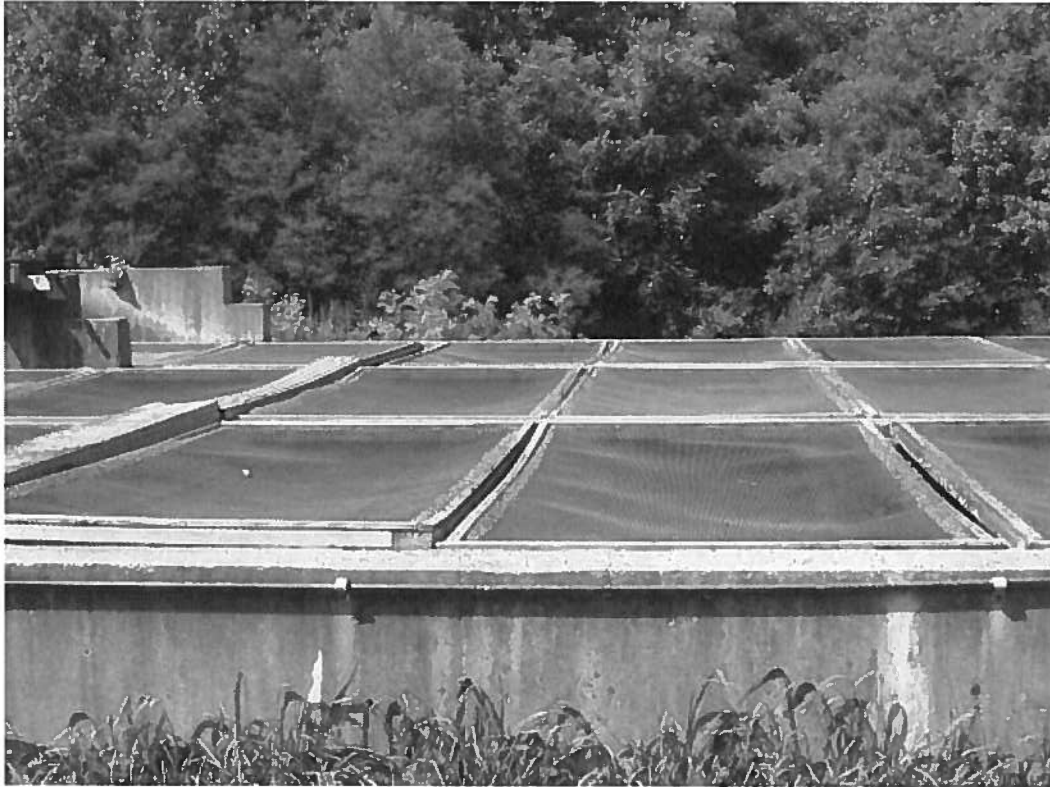
Figure 19. Plastic mesh in wooden frames helps to prevent entanglement, falls into the water, and bird depredation.
