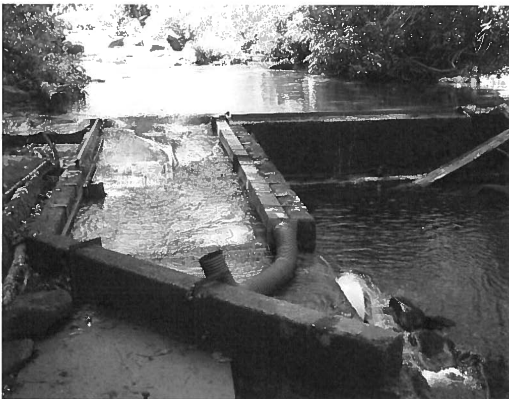
Figure 30. Trout farm head box in North Carolina bringing water from a mountain stream to the fish.
