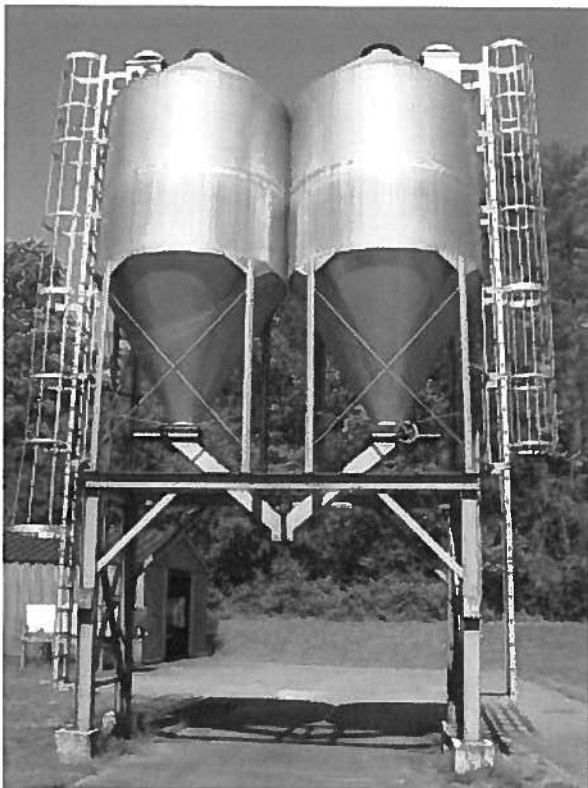
Figure 35. The ladder guards could prevent a fall if a worker slips from these feed bin ladders.
